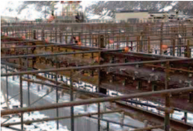
Fig. 8: Steel-panel bulkheads with horizontal corrugations were used as a form between sections
