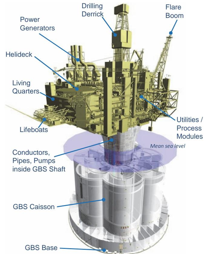
Fig.1 Hebron Oil Drilling, Production, and Storage Platform
