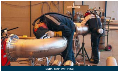
NMP - 6MO WELDING
