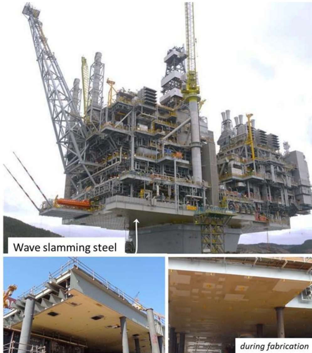
Figure 5—Wave Slamming Steel Underside of the Cellar Deck
